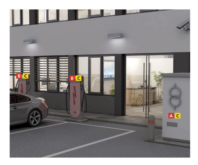
A storm is never planned and, what few electric vehicles owners and charging station operators know, charging posts require lightning and surge protection to prevent damage both to the posts themselves and the vehicle when charging during a storm.
