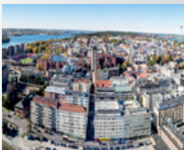
Residential & Commercial buildings - Tampere, Finland
